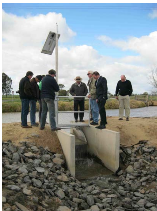
Inspecting the flood gate as it released water into the farm channel
