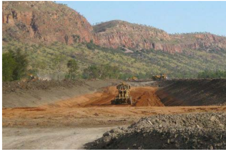
Construction of new roads and irrigation channels as part of Stage 1 of the Ord-East Kimberley Expansion Project
