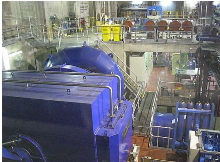
One of the turbines in the hydro electric power station
