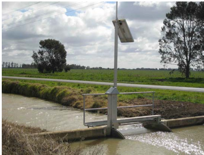
New flood gate in irrigation channel
