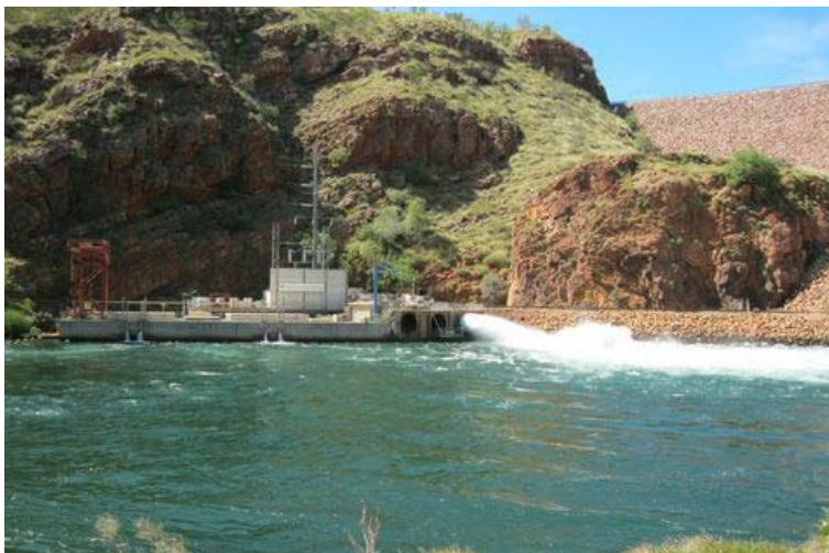
Ord River hydro electric power station
